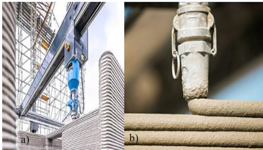
Figure 1 (a-b). 3D concrete printing in the construction application (source: googleimages)
